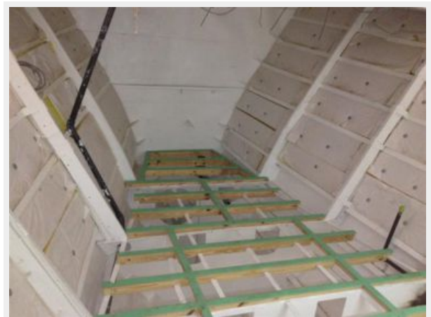
Floor Framing In Bow
