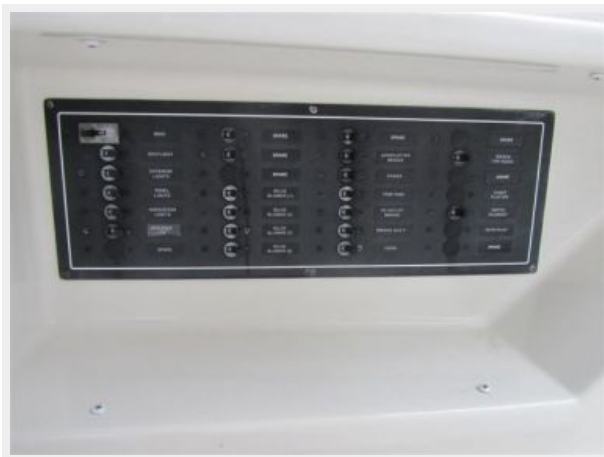
38' Carver electrical panel
