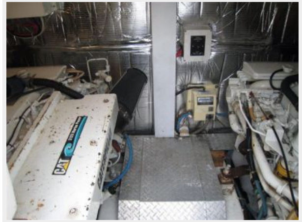
Door leading into engine room
