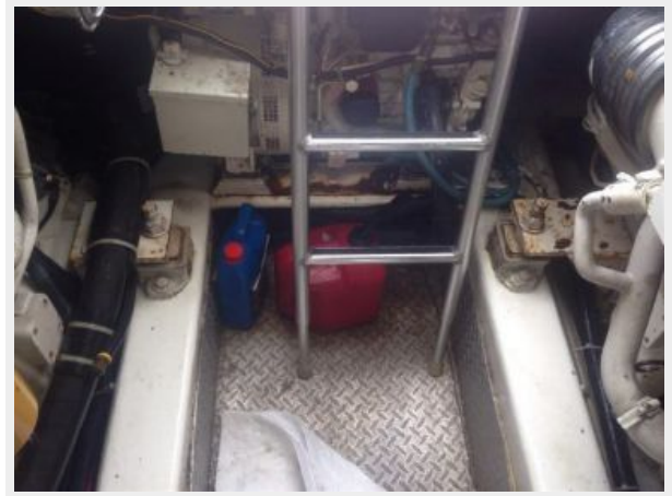
Generator in engine room
