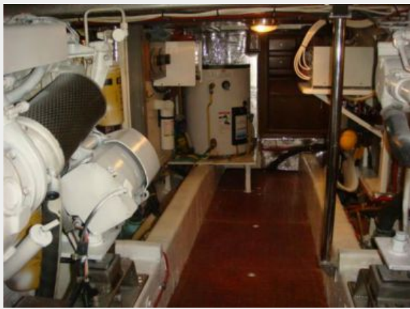
45' Ocean Alexander engine room forward
