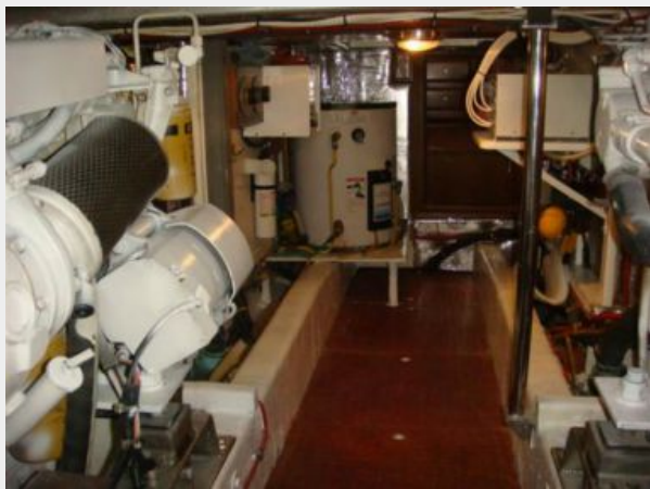
45' Ocean Alexander engine room forward
