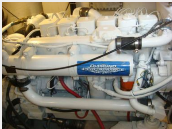
35' Tiara starboard main engine
