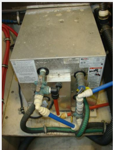
35' Tiara water heater
