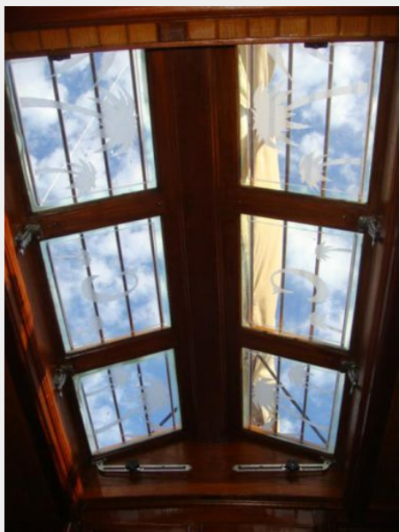
45' Coronado salon overhead deck hatch
