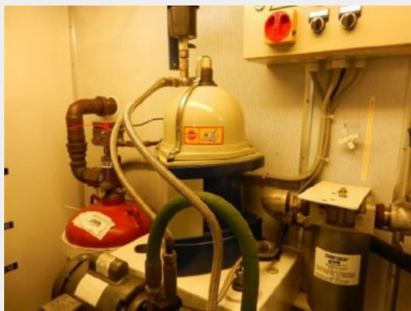
Alfa laVal Fuel Polishing centrifuge
