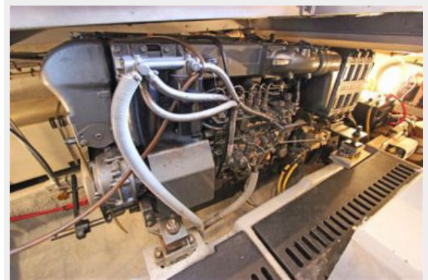
Starboard Yanmar Diesel Engine
