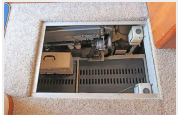
Salon Engine Room Access
