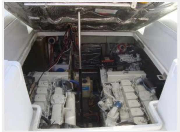
Engine Compartment - Under Bridge Deck
