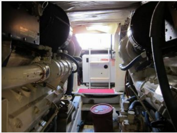
Engine room facing aft
