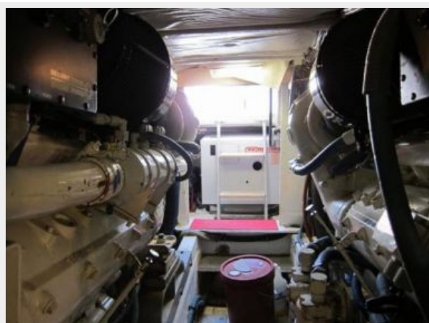
Engine room facing aft
