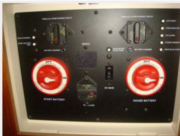
38' Hunter battery switches
