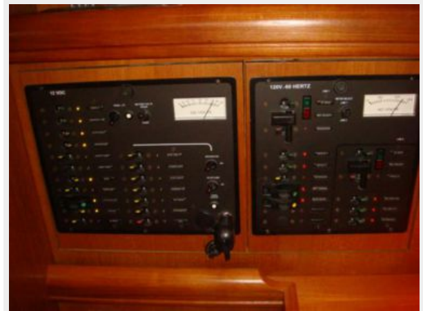
38' Hunter electrical panels
