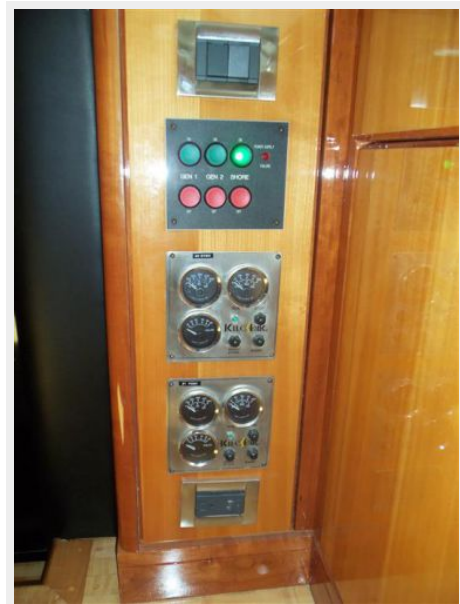
Pilothouse Generator Gauges
