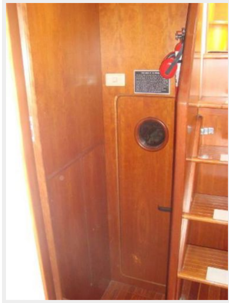
Entrance to Engine room
