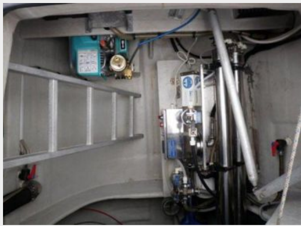
Starboard Machinery Space
