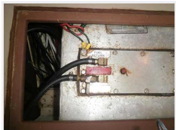
Fuel Tank Access
