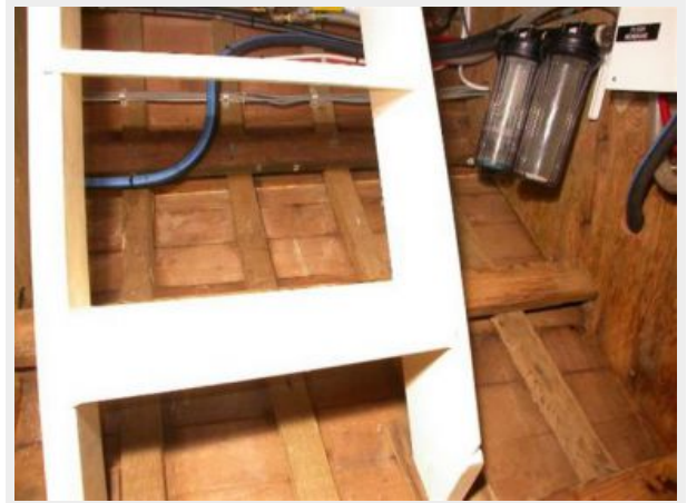
Stair to forward machine room
