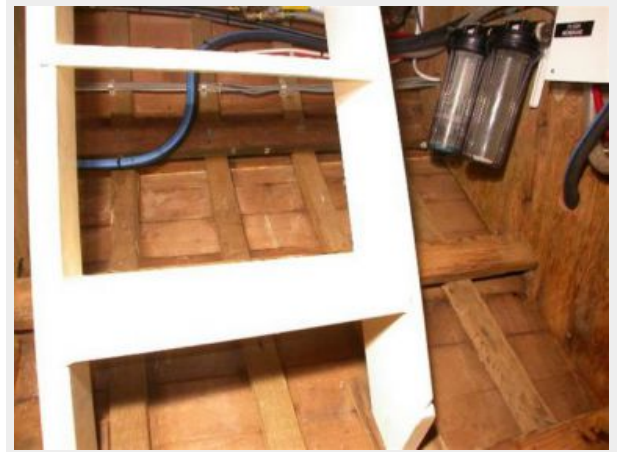
Stair to forward machine room
