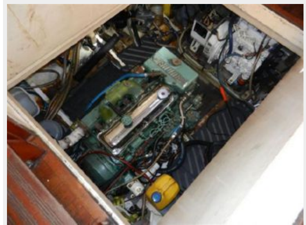
Engine access under floor boards
