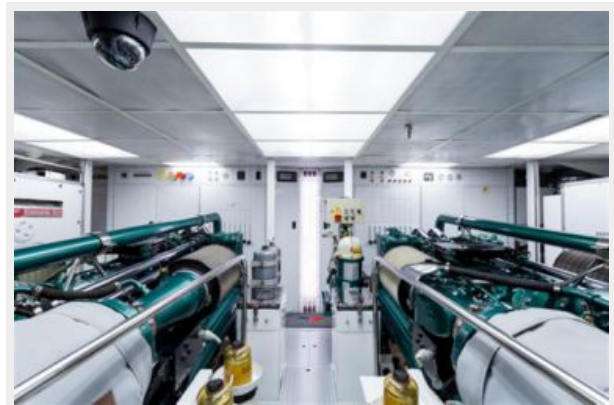
Engine Room Forward View
