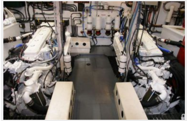
Engine Room - View Fwd
