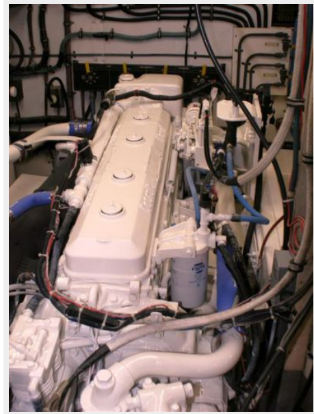
Engine Room - Stbd Main
