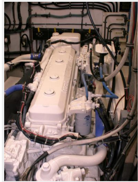
Engine Room - Stbd Main
