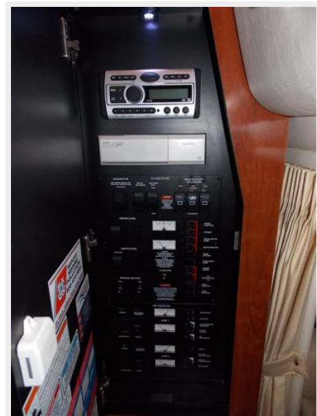
Main Distribution Panel
