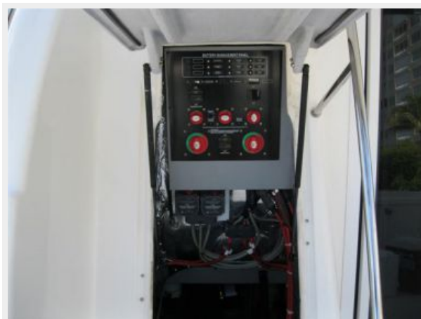
Engine Room Access
