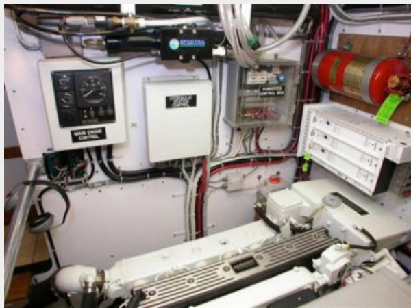
Engine Room detail 1
