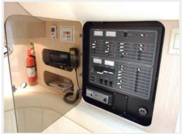
Electrical Panel Salon
