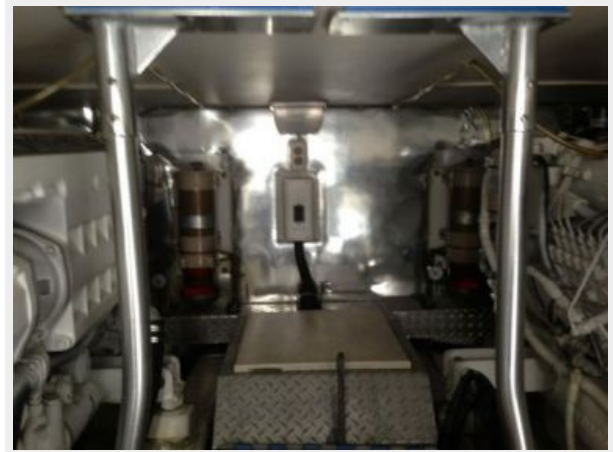
Engine & Mechanical Equipment 1
