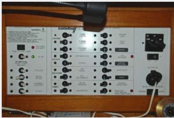
Main Breaker Panel
