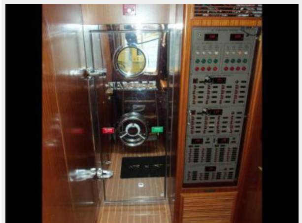
Engine Room Entrance
