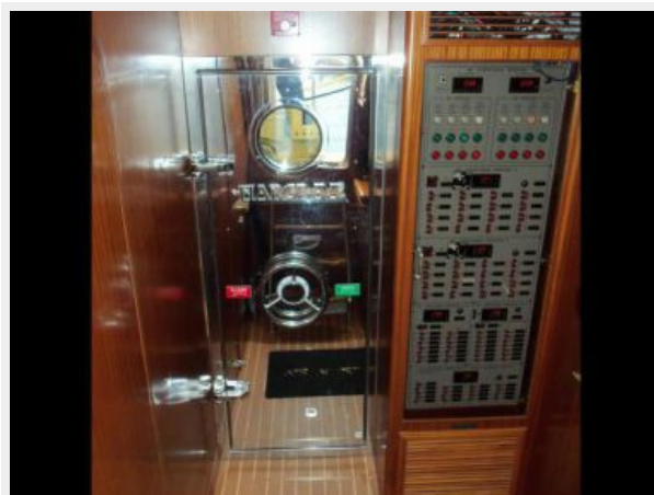
Engine Room Entrance
