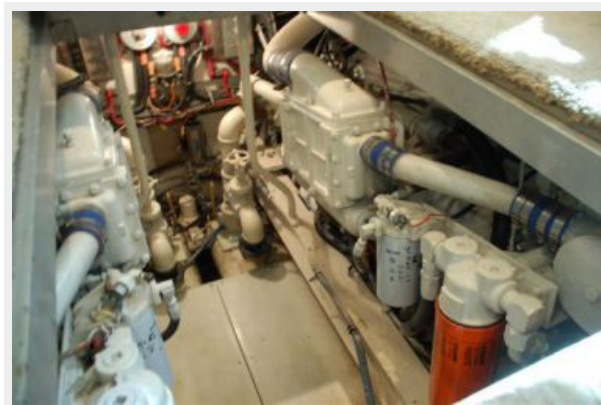
Engine room centerline
