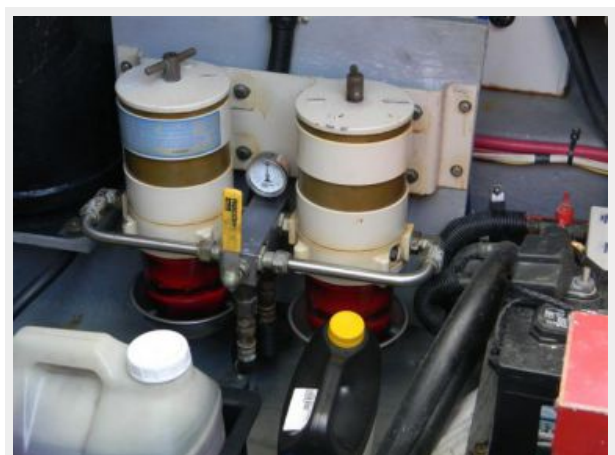
Racor Filters - Starboard
