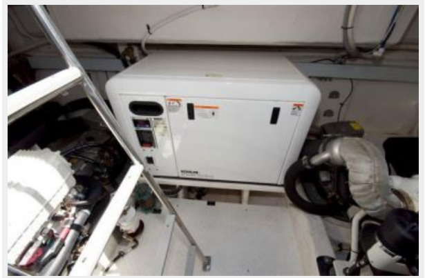
Engine Room- Generator
