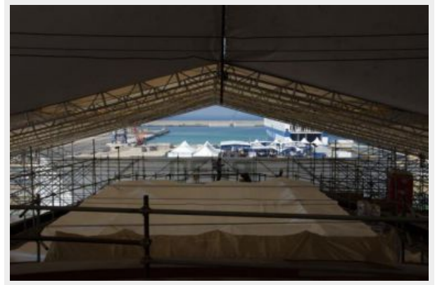
Under the Build Shed
