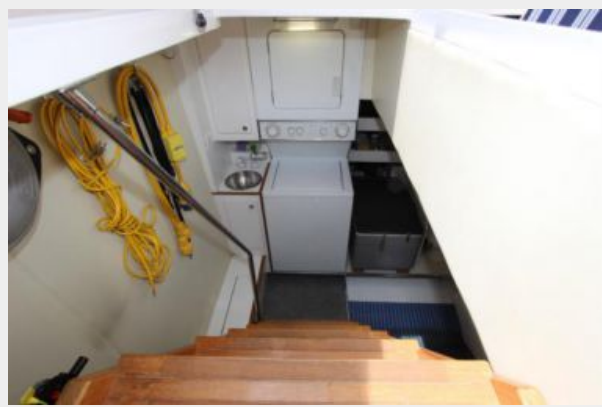
Engine Room and Crew Companionway
