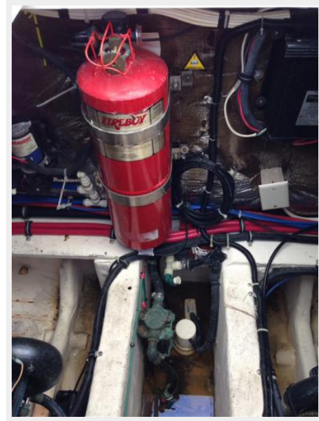
Engine fire suppression
