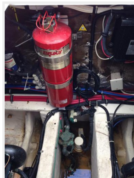
Engine fire suppression
