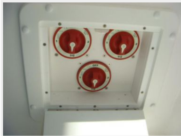
38' Renegade battery switches
