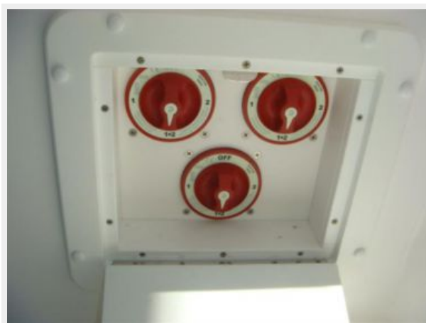
38' Renegade battery switches
