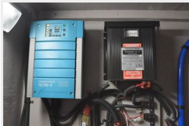
Upgraded Battery Charger in Utility Room
