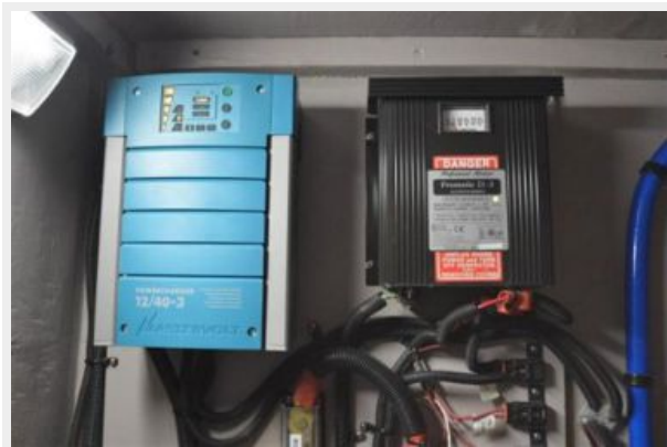
Upgraded Battery Charger in Utility Room
