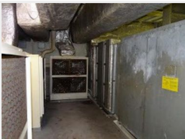
Air Conditioning Space
