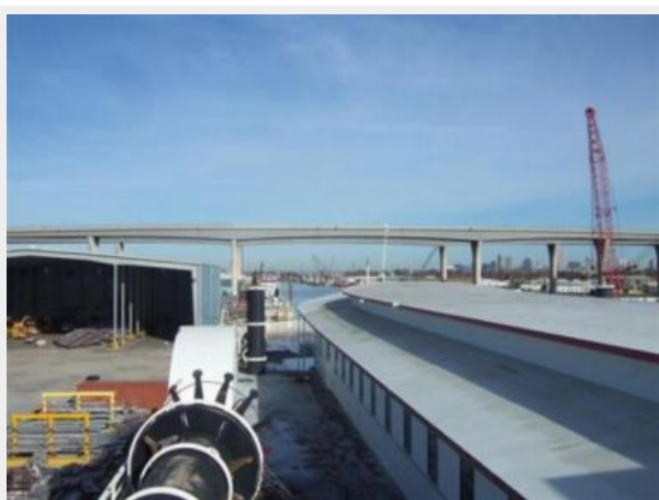
Starboard Side - Looking Aft
