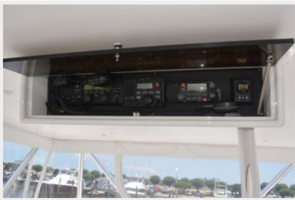
overhead electronics box
