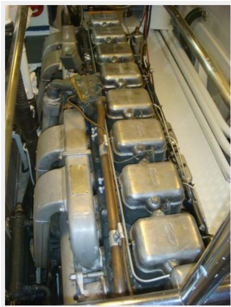
97' Santa Margherita port main engine photo2
