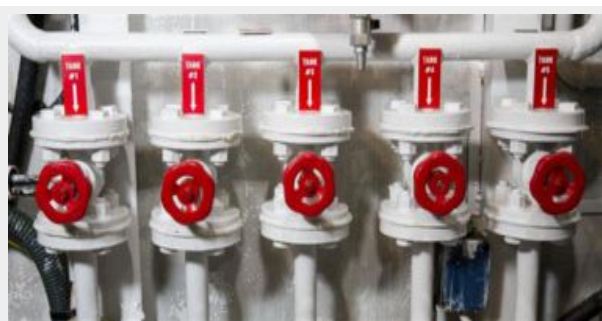
97' Santa Margherita fuel manifold
