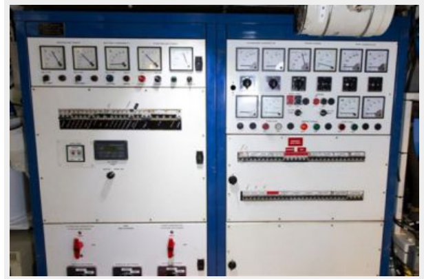
97' Santa Margherita engine room electrical panels
