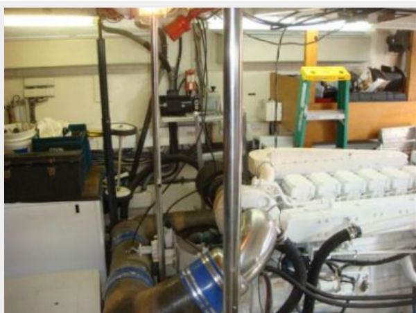
64' Hatteras engine room starboard
