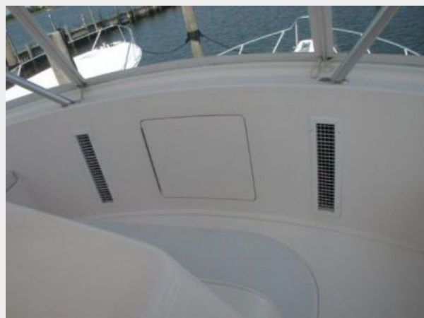
Deck 5 - Bridge Air Conditioning
