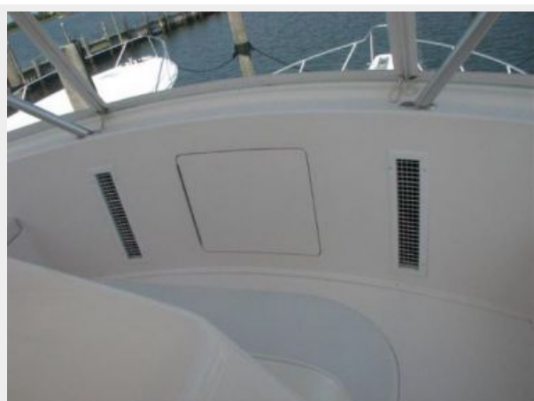
Deck 5 - Bridge Air Conditioning
